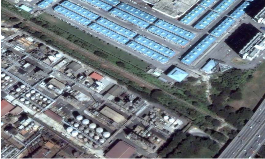
Picture 3: Chemical installation in urban areas and highways
